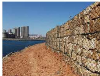
River Bank Protection
