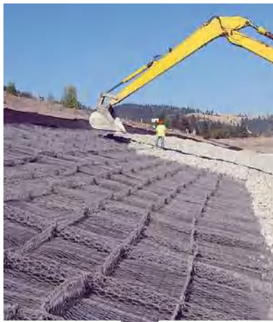
Soil erosion control
